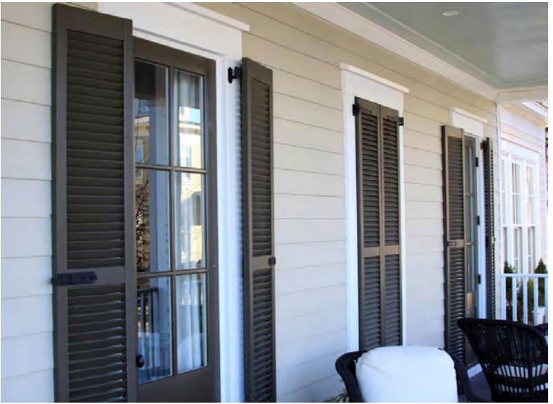
SHUTTERS. Shutters should be operable and sized to cover the opening they flank.
