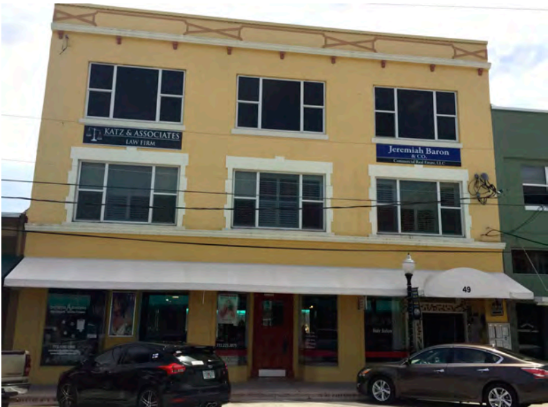
49 SW FLAGLER AVE. STUART, FL. A mixed use building with storefronts on the ground floor and an entry providing access to upper story offices. The facade is comprised of a three bays. Ornamentation is a simple cornice line between the first and second stories, an articulated parapet, and lintels over second story windows.
