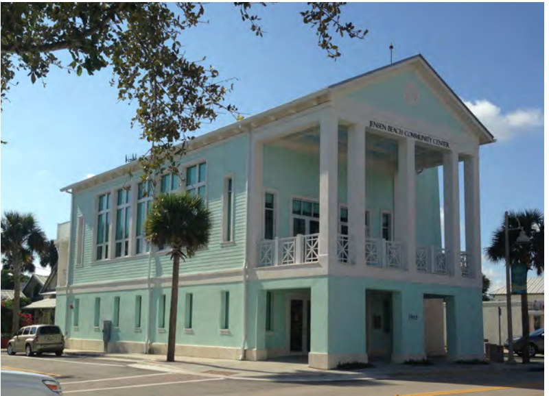
JENSEN BEACH COMMUNITY CENTER, JENSEN BEACH, FL. Constructed in 2010, the civic building provides a Classical example in the Florida Vernacular tradition. The stuccoed first story creates the building's base, with the upper story finished in siding. A prominent porch overlooks the street, expanding the main congregational space in the second story.
