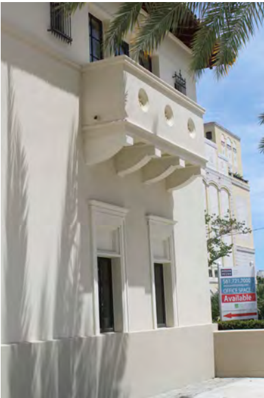
COMMUNITY FOUNDATION, WEST PALM BEACH (LEFT) & WORTH AVENUE, PALM BEACH (RIGHT). The scale of the brackets respond to the visual weight of the balconies: the “heavier” balcony with the solid wall enclosure (left) is supported by four large brackets; the balconies on the right, with thin floors and light metal railings, are supported by iron scrollwork.
