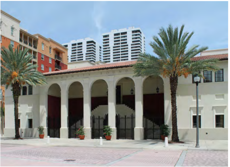
COMMUNITY FOUNDATION, WEST PALM BEACH, FL. This building, designed in the Classical Tradition by Portuondo Perotti Architects and constructed in the early 2000s, has a clearly articulated base, central mass, and top. Classical detailing is expressed in the double-height loggia, bracketed masonry balconies, and a symmetrically balanced facade.
