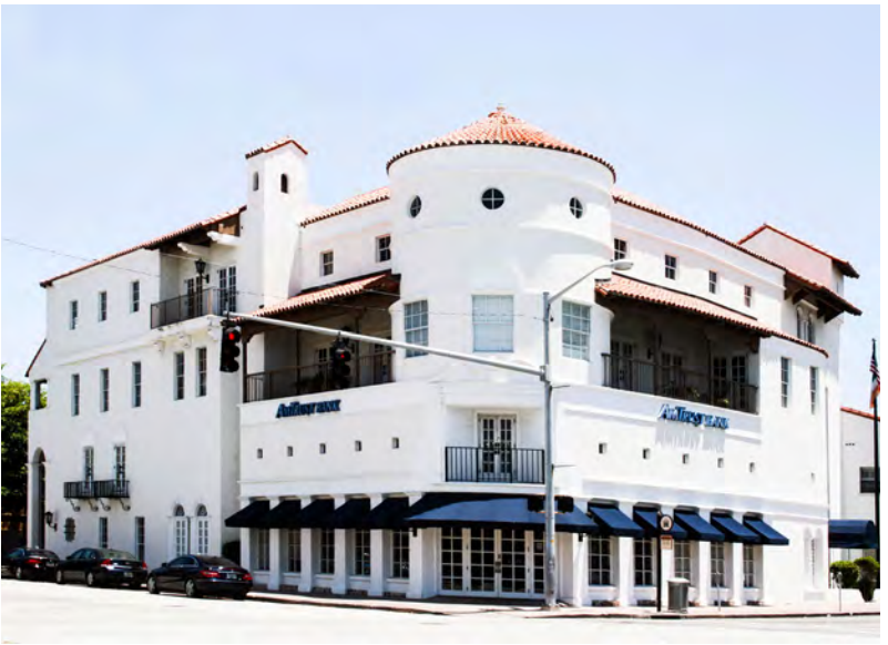
AM TRUST BANK, CORAL GABLES, FL. This building has a variety of compositional devices, including loggias and balconies, that reduced the visual scale of a relatively large building. The significant outdoor spaces within the mass of the building are all covered - an important characteristic in the Florida environment.
