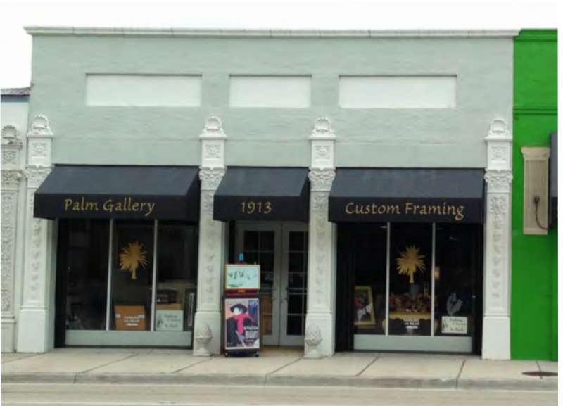
1913 S. DIXIE HIGHWAY, WEST PALM BEACH, FL. This shop illustrates the type of ornamental friezes and pilasters that were frequently incorporated in the 1920s. Buildings remain simple in form with decorative elements typically applied between bays, around openings, or within parapets.
