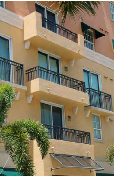
MIXED USE BUILDING (LEFT) & COMMUNITY FOUNDATION, WEST PALM BEACH. The brackets on the building on the left are too small for the balconies they “support”. Smaller corbels are appropriately used to support a balustrade (right). Also, the upper balcony interrupts the cornice line; better compositions are shown in the top right and left images, which incorporate the cornices into the detailing.
