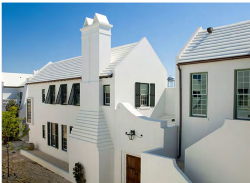
57 GOVERNORS COURT, ALYS BEACH, FL. Anglo-Caribbean architecture typically elaborates and sculptural shapes masonry elements. Generally this detailing occurs on the parapets, chimneys, entries, and stairways.
