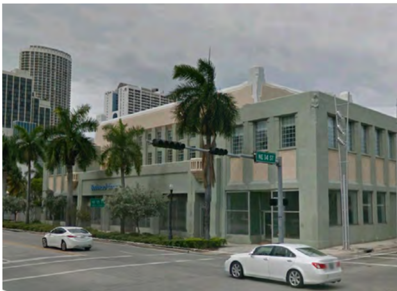
OFFICE BUILDING, MIAMI, FL. This Art Deco example has a three-story central mass, and two-story wings. Art Deco motifs including articulated parapets and corners decorate a fairly simple geometric massing. At ground level, large store-front openings help provide visual interest for pedestrians.
