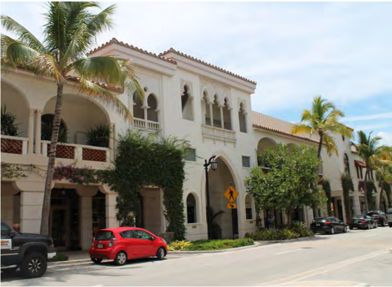
150 WORTH AVENUE PALM BEACH, FL. This mixed use commercial building has a multi-levelled parking garage integrated into its design; however, the variation of heights and the use of arcades and loggias and an interior courtyard help break down the mass and make the building compatible in scale with the surrounding context.
